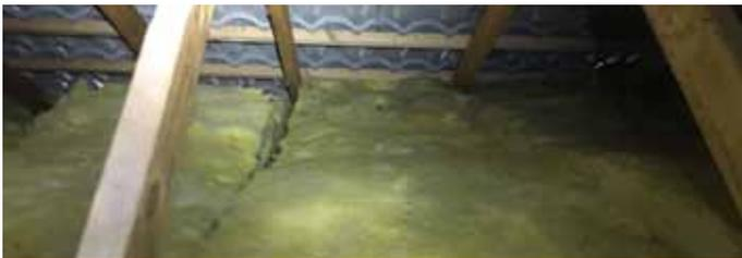
R6 insulation installed correctly in most places
