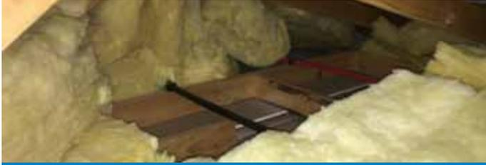
A number of areas were identified that were missing insulation. These will be rectified by the builder.
