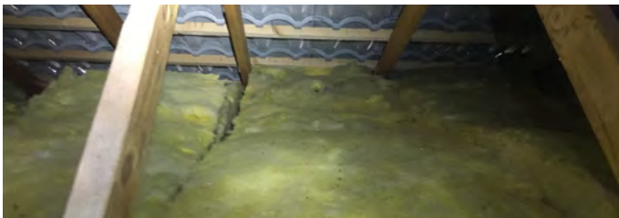
R6 insulation installed correctly in most places
