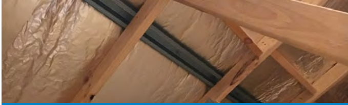
Anticon Blanket R1.3 under colorbond roof. As well as assisting insulate the home it stops condensation and dust entering the roof space.
