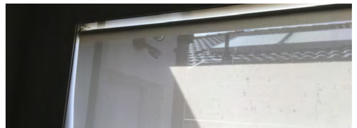
Installed a number of smaller windows to east and west
