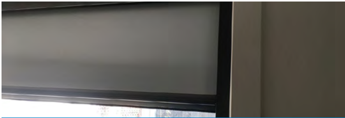
In many rooms window sizes were reduced and screen away blinds installed to block radiant heat from the sun.
