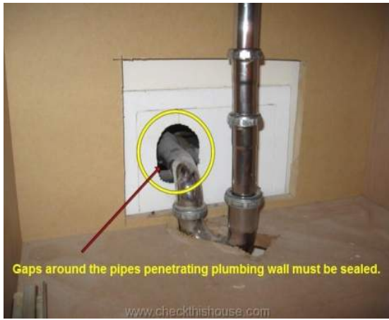
Sealing plumbing holes
