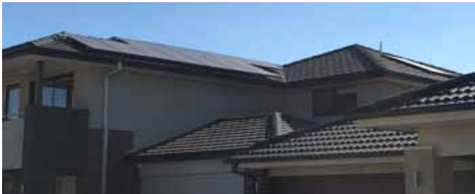
6.2kw Solar System
